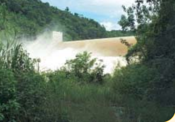
BECOL owns and operates the Mollejon hydroelectric facility located on the Macal River.
